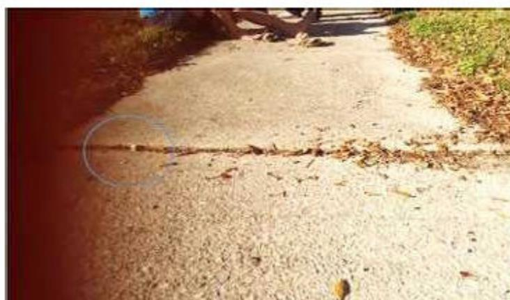
More than two-and-a-half years after the fall, Jackson's retained engineering expert inspected the sidewalk. He opined that the uneven sidewalk constituted a tripping hazard because the vertical misalignment at the expansion joint was greater than  $\frac{1}{2}$  inch. In forming his opinions, the expert relied on numerous standards and regulations, including, *inter alia*, the Florida Building Code.
